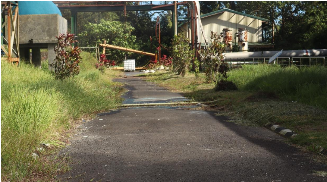
Gambar 9. Area Belakang Cooling Tower II
